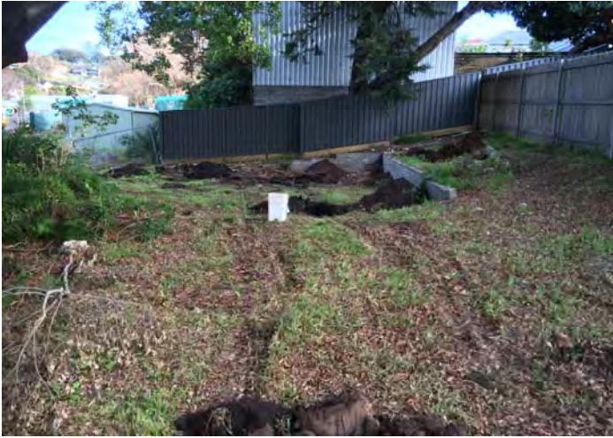
Plate 1 (30 June 2016) View of rear yard at 104 Shoalhaven Street, Kiama. The retaining wall marks the area of the former transpiration bed. Several testpits (TP-2 & 3 and 5) are visible at the centre of the frame and location of transpiration bed. Plate 2 showing the aged fibro and brick constructed house and front yard. Plate 3 viewing east over the side driveway and location of BH-1 (next to yellow bin). Plate 4 showing the rock wall and stormwater drain on the southern boundary. Plate 5 showing the fibro garden shed located on the rear yard and south boundary.
